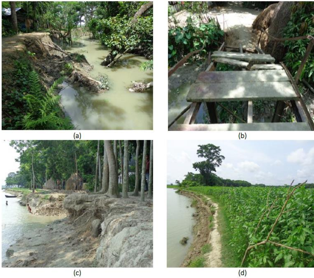
Figure 12. Impacts of natural disasters on soil, infrastructure, forest, and agricultural land in Kazirchar village, (a) soil erosion, (b) damage to main road to village entrance, (c) losses of homestead forest, and (d) losses of agricultural land.
